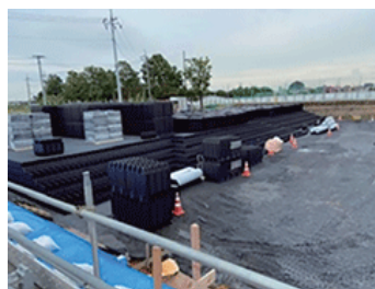
Construction of the storm water detention tank
