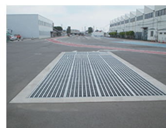
Flood prevention measure (drainage grid) (Utsunomiya Plant)
