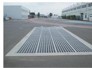
Flood prevention measure (drainage grid) (Utsunomiya Plant)
