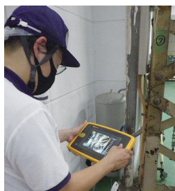
Air leak investigation
