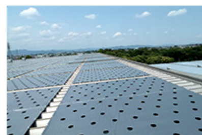
Insulation sheets attached to a plant roof
