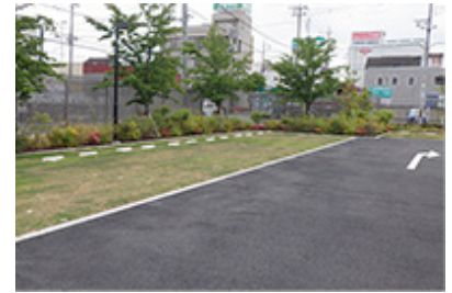
Car park with a flood prevention measure (Gunma Plant)
