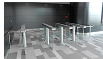
Entry and exit gates through which people in wheelchairs can also pass at the new West Main Building at the Gunma Plant
