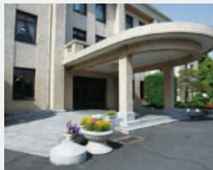
The main building at the Gunma Main Plant provides accessibility with wheelchair ramps
