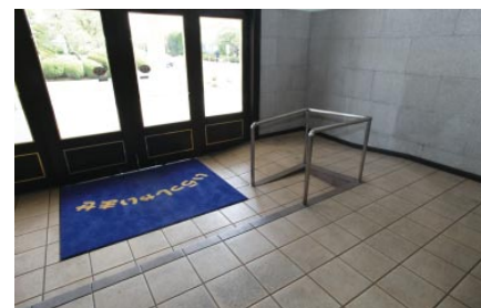
Wheelchair ramp installed in the entrance of the main building of the Gunma Main Plant
