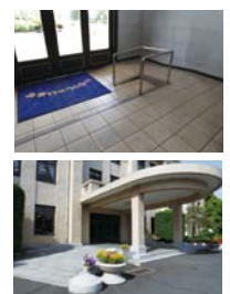
Slope installed at the manufacturing facilities
