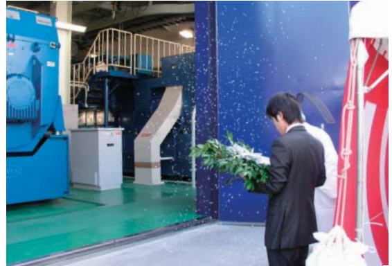
Cogeneration start-up ceremony at the Oizumi Plant
