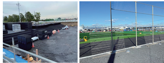
Construction of the storm water detention tank | Donated tennis courts
